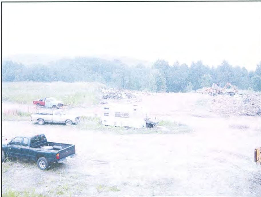
Photo 12. Disturbed - C&D Landfill
